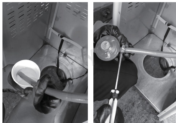
Correct connection of the hose and regulator to the gas cylinder.
